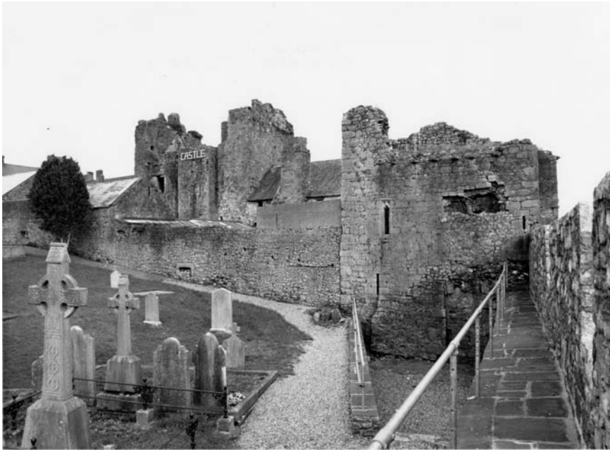
Figure 1. Medieval buildings on the east side of the churchyard in Fethard, county Tipperary: “Fethard Castle” is centre-left; a second building of c.1500, called “Edmond’s Castle”, is on the right.
